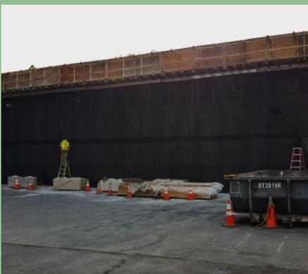
Hanging Debris Net Against Shoring Towers at the Cantilever Edge
