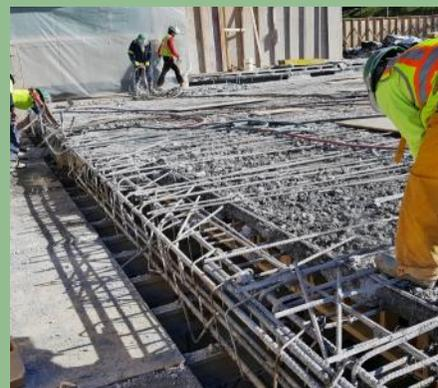
Full Beam Replacement at the Cantilever Edge
